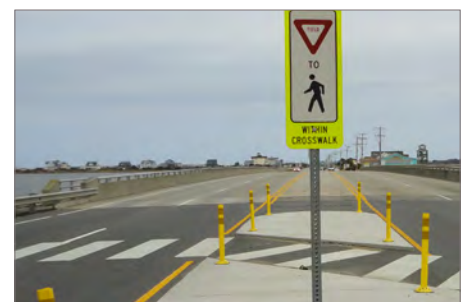
Pedestrian crossing with high-visibility crosswalk, raised median island, flexible bollards, and signage (near the Little Bridge Fishing area).
