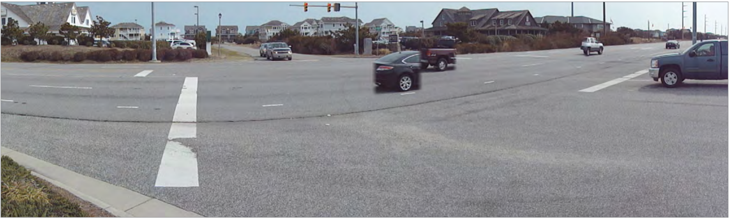
Lack of Connectivity Example: Looking east across US 158 down E. Epstien towards the beach. There is no crosswalk or pedestrian signal connecting pedestrians from the beach and municipal buildings on the east side, to Food Lion and the shopping areas on the west side.
