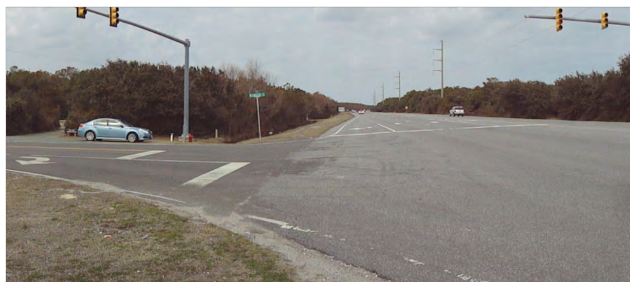
Looking north along US 158 from Carolista/Hollowell. The future path run between US 158 and the trees/vegetation shown in this photo. If right-of-way allows, the trail should meander through the trees for shade. Crossing improvements would include high-visibility crosswalks and countdown signals for the trail.
