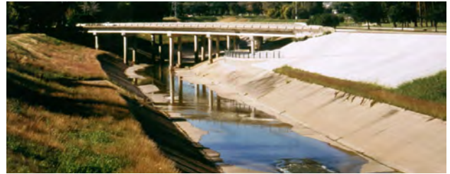
Trails in river and utility corridors
