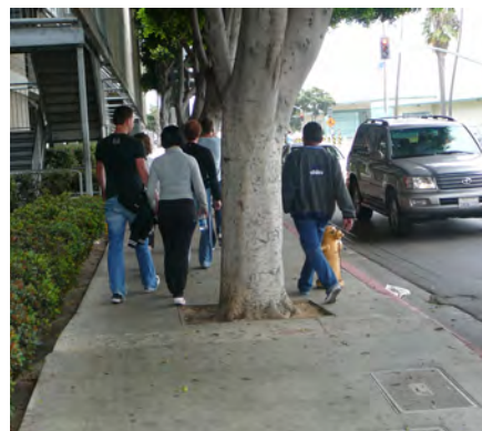
Sidewalk obstructions and driveway ramps
